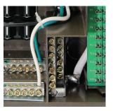
Built in terminal bars for the negative DC wiring eliminates the time and cost of installing a separate negative DC bar.
