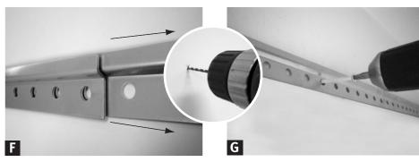
Extend second hang rail Slide second hang rail as far right to the wall as possible while still maintaining hole alignment. Repeat step **C** to secure to the wall. If there is **not** a stud within 4" of the RIGHT end of the hang rail, repeat the dry wall anchor installation step above.
