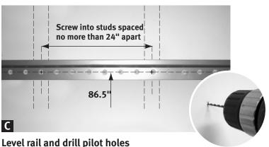
Level hang rail and mark holes 86.5" above floor that land on studs, then drill 1/8" pilot holes for screws.
