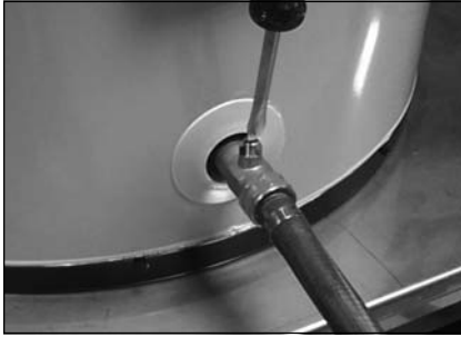
Draining the old water heater.
