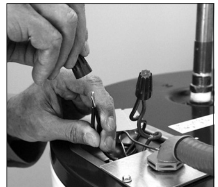
Figure 19 - Connecting the electrical wires.
