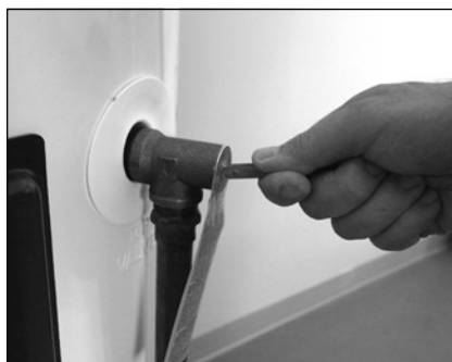
Figure 38 - T&P Relief Valve
