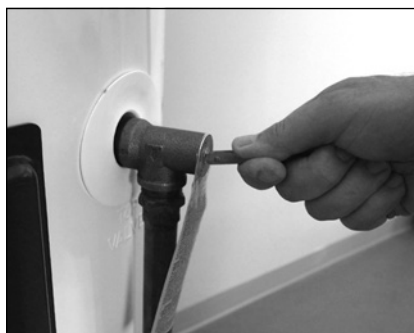
Figure 38 - T&P Relief Valve
