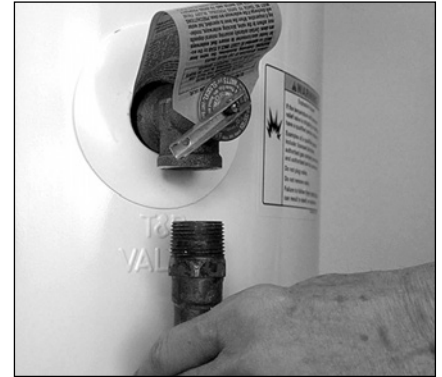
Figure 21 - Removing the T&P Relief Valve discharge pipe.
