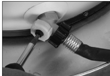
Figure 20 - Draining the old water heater.
