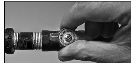
Figure 58 - Gas valve in “on” position.
