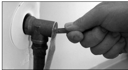
Figure 45 - T&P Relief Valve.
