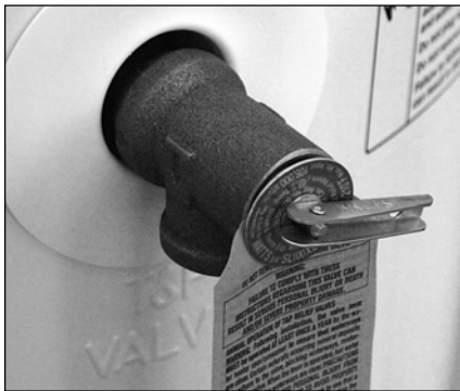
Figure 25 - Temperature and Pressure Relief Valve
