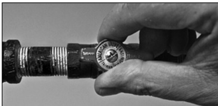
Figure 32 - Gas valve in "on" position
