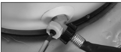
Figure 42 - Draining the water heater.
