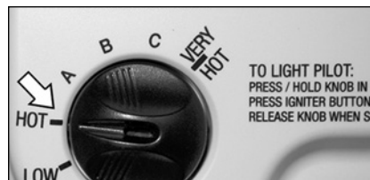
Figure 36 - Adjust the gas control knob to "HOT".
