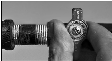
Figure 50 - Gas valve in “off” position.
