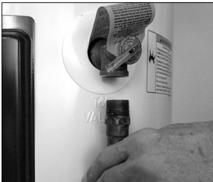
Figure 11 - Removing the T&P Relief Valve discharge pipe.
