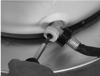
Figure 10 - Draining the old water heater.
