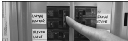
Figure 24 - Circuit Breaker
