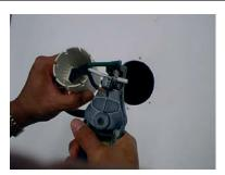
3. Strip wire ends 1/2" to 5/8". Make sure the wire strands are clean and not corroded. If necessary, cut back the wire until clean wire is uncovered. not solder the ends of the wire.
