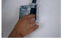
2. Unscrew strain relief to release cable It may be necessary to replace with ded strain relief. Pass the cable provided strain relief. through strain relief and box extender.
