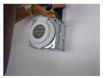
6. Position the gasket and inlet over the box cover opening, align the mounting holes and attach the inlet with provided 8-32 screws. It may be necessary to pull cable back out of the box through the strain relief to prevent wires from crowding. Fasten the box cover to the box extender and tighten the strain relief to 12-16 in.-lbs. torque.
