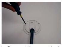
1. Remove existing mouse hole plug housing by unscrewing three mounting screws. Pull out and cut off cable leaving enough cable from the mounting hole to work on (approximately 12 to 18 inches).
