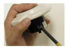
4. Back off terminal screws on the rear housing of the inlet. Insert wires into color coded openings on the back of the inlet. Tighten terminal screws to 14-20 in.-lbs. Make certain there is no wire insulation under any terminal and the gasket is in place. Note: Two gaskets provided, use the gasket that best fits your installation
