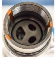
1. View the 1255 cartridge to find the three small tabs protruding. Look into the chamber of the faucet to find the location of the three large grooves. The grooves will accept the small tabs protruding from the 1255 cartridge. These tabs and grooves are highlighted in orange above for demonstration, but will not be orange on your cartridge and faucet.
