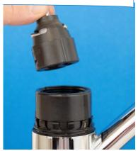
Insert the 1255 cartridge into the chamber making sure to line up the three tabs with the grooves.
