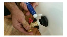
12. Screw in the discharge valve and quarter-turn inlet valve as shown. Tighten by hand only.
