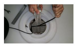
5. Remove the zip tie and the bolt & nut in the center of the pump mount.
