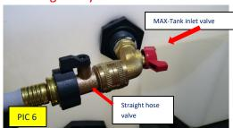
**Step 6:** Switch on the pump and allow a few seconds for the pump to self-prime. **DO NOT allow the pump to run dry for any prolonged period of time.**
