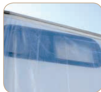
Plastic sheeting protects the sidewalls.
