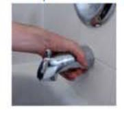
Turning counterclockwise, remove the old Tub Spout. If your Tub Spout has a set screw holding it in place, be sure to remove that prior to rotating the Spout off. If your Tub Spout is hard to remove, you may need to use the end of a hammer or large wrench to help loosen while turning. Just insert the handle into the opening of the Tub Spout for leverage.
