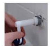
Turning clockwise, apply 6 to 8 turns of the Pipe Thread Tape to the threads on the Male end of Extension Nipple.
