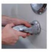
Turning clockwise, tighten the new Spout onto the Extension Nipple.
