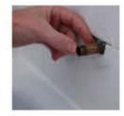
Measure the Stub Out Nipple length from the wall surface to the end of the Pipe. The Stub Out Nipple must be between 2" and 3" long. The end of the Stub Out Nipple should be even.
