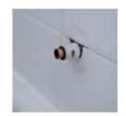
Slide the O-ring onto the Stub Out Nipple at least 1/2" from the end of the Nipple.
