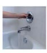
Turn water on and test for leaks. If water is leaking from the rear of the Tub Spout, reinstall, as this could damage your wall.
