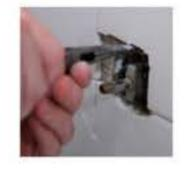
Remove the Retainer Clip carefully as not to drop it behind wall.
