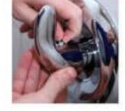
The easiest way to remove the old Cartridge is to use a Cartridge Puller. Make sure to follow the instructions for the Cartridge Puller, which can be purchased at your local home improvement store. Because Cartridges are unique to specific type of Faucets, you will want to take your old Cartridge to your local home improvement store and use the Perfect Match locator system from Danco or use the online Stem Finder. This system makes it easy to find your replacement.
