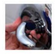
Slide the Handle onto the Stem or Handle Adapter onto the Stem. Do not use Handle Screws at this point. Turn the water supply back on and test for leaks and ensure the hot water temperature is adequate. Be sure not to exceed the maximum temperature allowed by local plumbing code. Finally, secure the Handle with the Set Screw and your project is complete.
