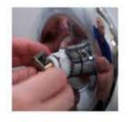
Reinstall the Retainer Clip, Stop Tube, Key Stop, and the Temperature Limit Stop, in that order.
