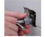
The easiest way to remove the old Cartridge is to use a Cartridge Puller. Make sure to follow the instructions for the Cartridge Puller, which can be purchased at your local home improvement store. Because Cartridges are unique to specific type of Faucets, you will want to take your old Cartridge to your local home improvement store and use the Perfect Match locator system from Danco or use the online Stem Finder. This system makes it easy to find your replacement.
