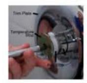
Next, remove the Temperature Limit Stop, Key Stop, Stop Tube, and the Trim Plate (as needed to access Cartridge).
