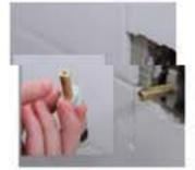
Insert the new Cartridge, Hot inlet Left Side, Cold inlet Right Side into the Valve Body with the tab stamped "HC" on top and with the Stem Notch down.
