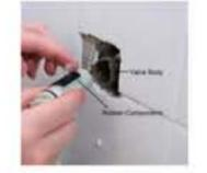
Using Silicone Grease, lubricate the inside of the Valve Body about 1". Then lubricate the Exterior Rubber Components on the Cartridge with Silicone Grease as well.
