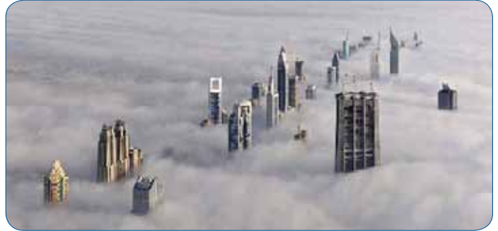
The tallest building in the world, the Burj Dubai, is one of several buildings in Dubai that has tapped Culligan to handle its Industrial water treatment needs
