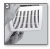
Squeeze grille springs, insert springs into fan slots and push new grille up against ceiling.
