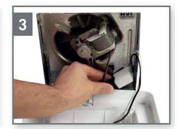
Attach second grille spring to fan and push grille up against ceiling.
