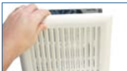
Remove the old grille and unplug the motor.
