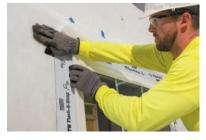
ance requirements that allow it to be left exposed up to 180 days, the self-adhering flashing features a treated release film on its adhesive side. Joining the company's extensive waterproofing solutions, the flashing comes in 4-, 6- and 9-inch rolls that fit a range of projects.
