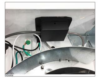
Install a momentary contact switch at a convenient place for the user. Connect the end of the provided ADA cable to this switch as shown below:
