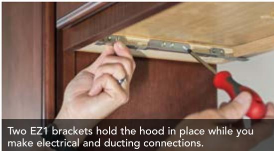
Two EZ1 brackets hold the hood in place while you make electrical and ducting connections.
