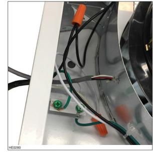
Strip the end of the 3 wires from GREY cable (the one with ferrite), then using small UL approved wire nuts (suitable for 22 AWG wires), connect these wires with ADA cable wires. Connect as follow: WHITE wire with WHITE wire, BLACK wire with BLACK wire and RED wire with RED wire.
