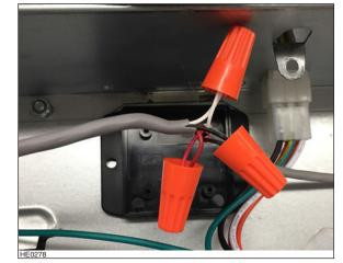
Put the wire nuts inside the connection box base, then snap the connection box lid on its base, ensuring the ADA cable runs through the open notches.
