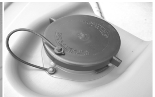
3" cap with strap attached--top of tank
