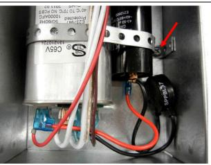
Place start capacitor next to run capacitor and secure with existing mounting strap (note: use other screw location as indicated by arrow).
