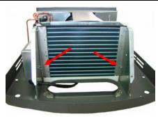
1. With the AC on a flat surface, remove outer shroud.
